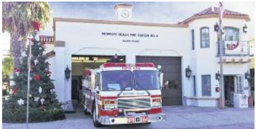
Present day Balboa Island Fire Station No. 4
